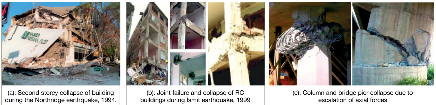
Fig. 1: Damage to structures caused by the vertical component of earthquakes
